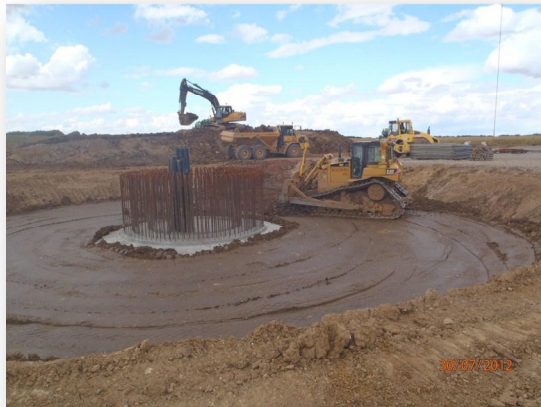
Duct Installation into turbine foundation.
