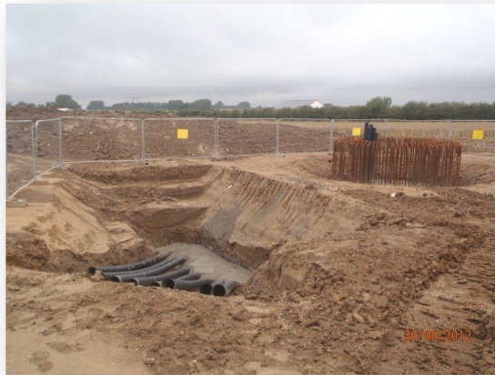
Duct Installation into turbine foundation.
