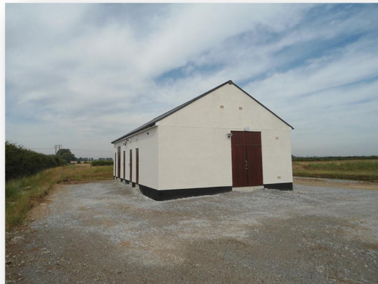
Substation – Complete awaiting fencing
