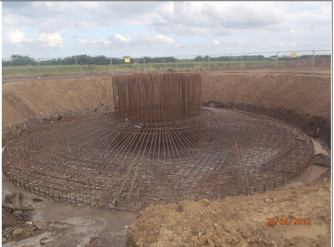
Turbine 9 reinforcing cage.
