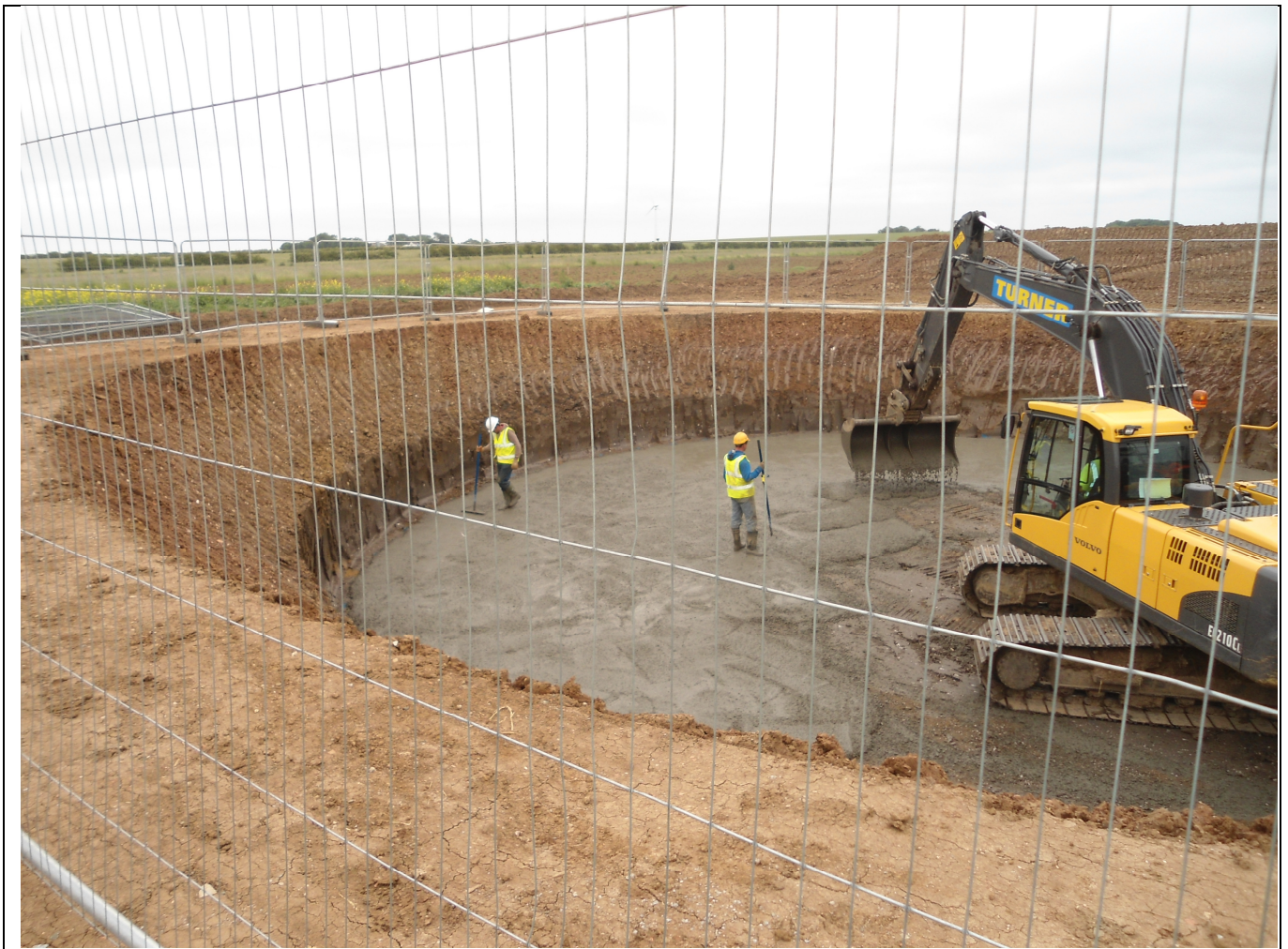
Placing Blinding to Turbine 2.
