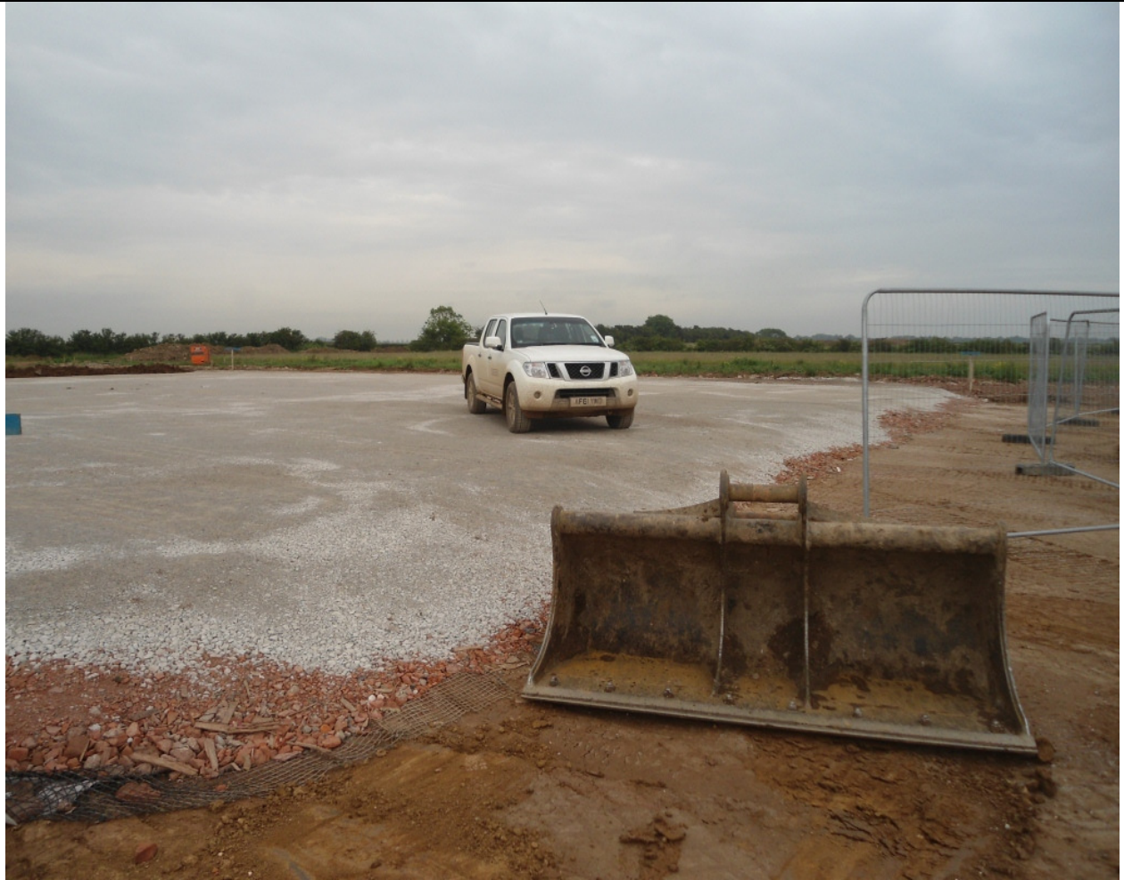
Crane Pad at Turbine 2
