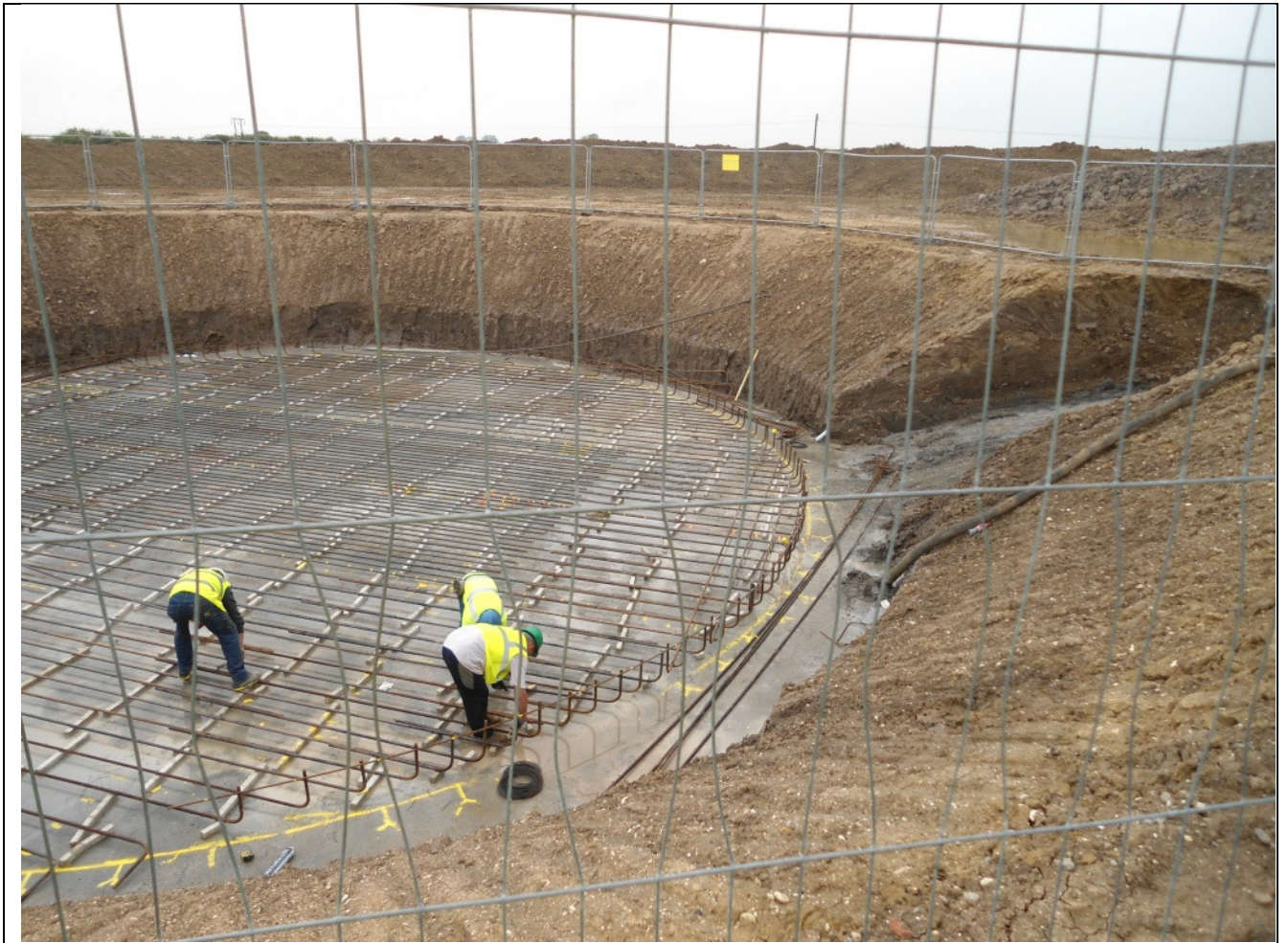
Start of Steelfixing at Turbine 3.
