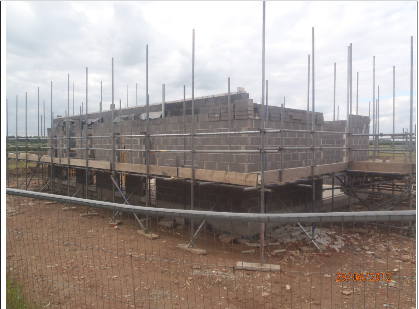
Substation Internal walls to wall plate level.
